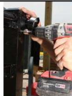
Fixed (wall) Mount Fitting – Mounts on post or other vertical surface. (Not available for Midway)
